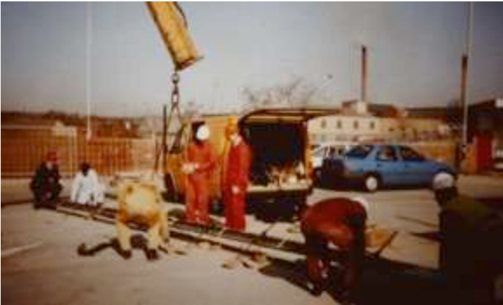
Rail lowered into beam
