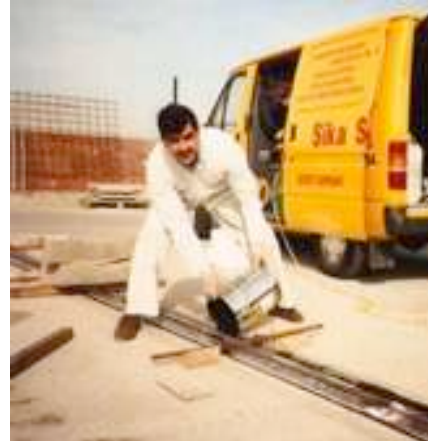
Rail bonded into beam
