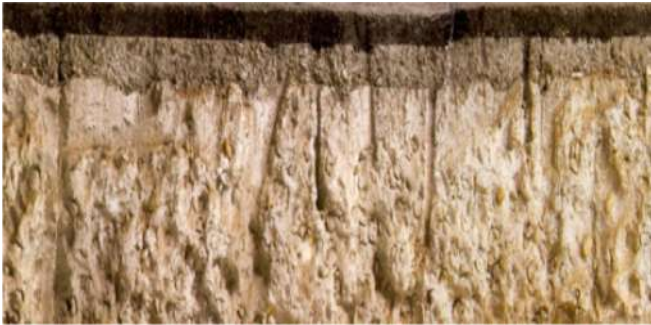
(1). Existing strong road pavement
